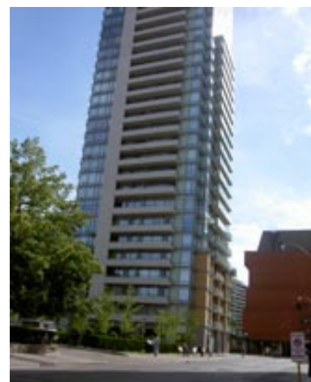
Typical "Tall Building".
